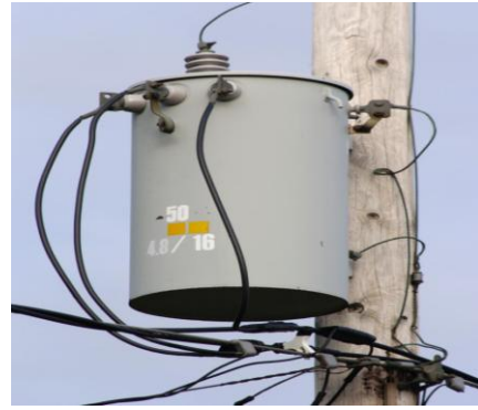
Electric pole transformer.
