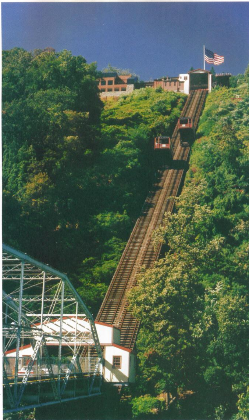
The Johnstown Vehicular Incline
