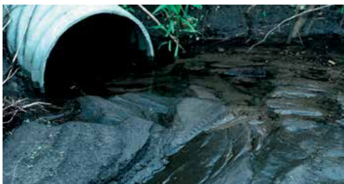
Sediments have filled up the opening of this drainage pipe that empties a stream into a lake.
